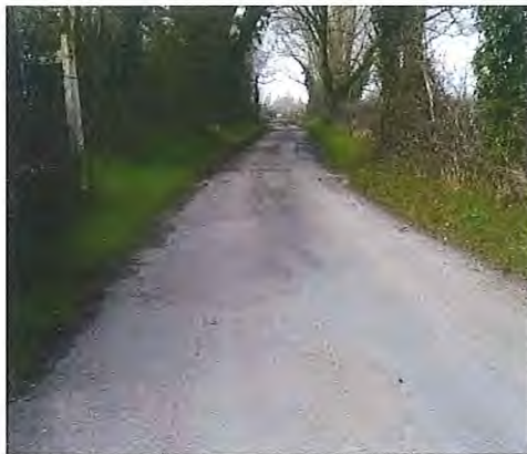
Church Road, looking West
