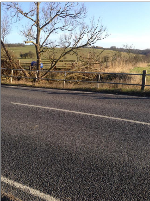
Figure 1 – B1010 Lower Burnham Road – View from Eastbound Lane
