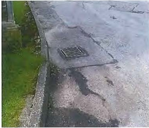
Existing gully located outside 'Old School House'
