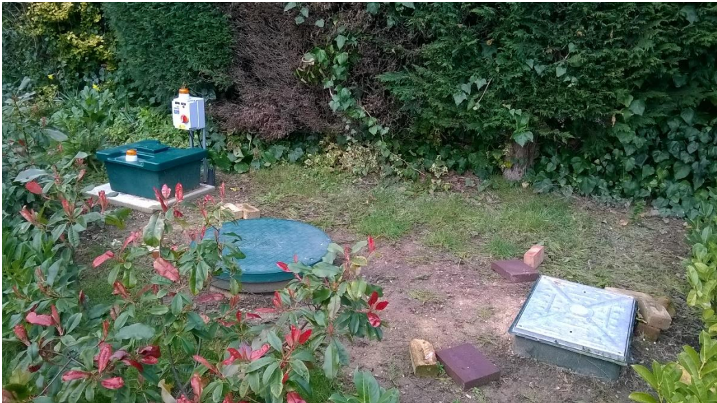
Cesspit in No.1 Little Mill Cottage front garden that services all four properties
