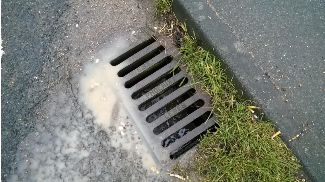
Gully in bell mouth of gated entrance to Doe's yard west of No.1 Little Mill Cottage (Gully 7 on CCTV survey)
