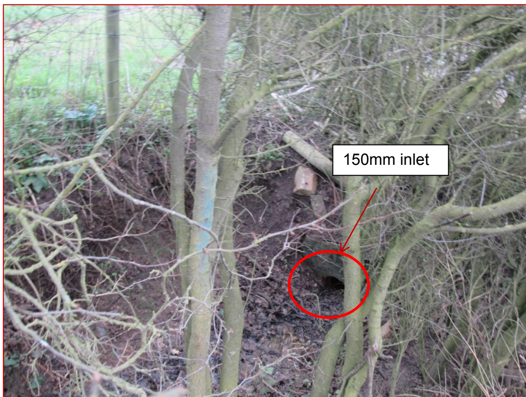
Figure 8 – Headwall / 150mm pipe at bottom of Martin's Lane (east side)
