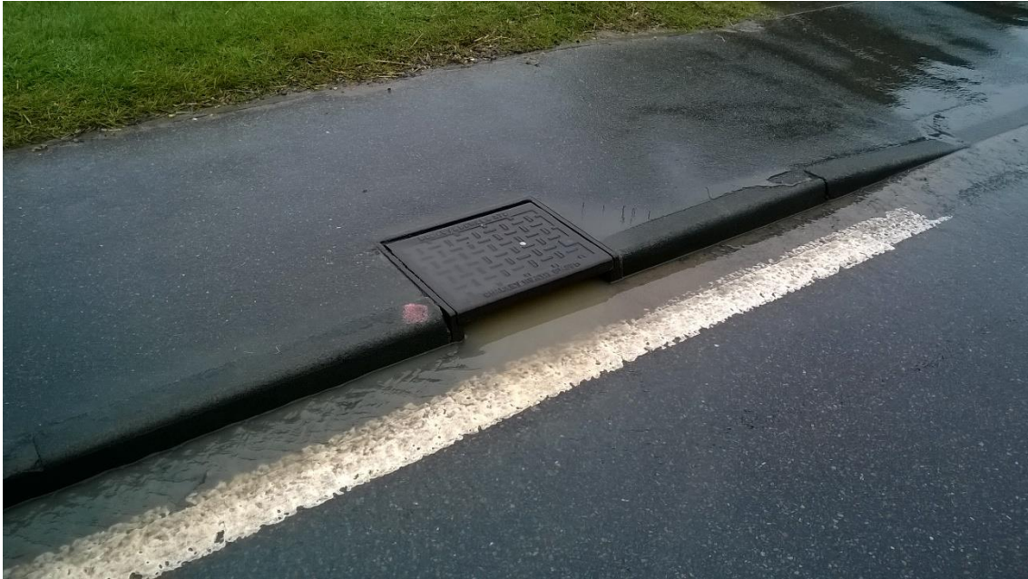
Kerb gully opposite No.1 Little Mill Cottage (Gully 6 on CCTV survey)
