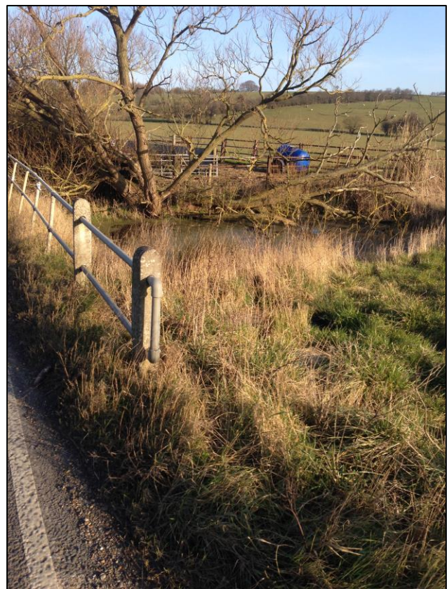
Figure 2 – B1010 Lower Burnham Road - Eastward View
