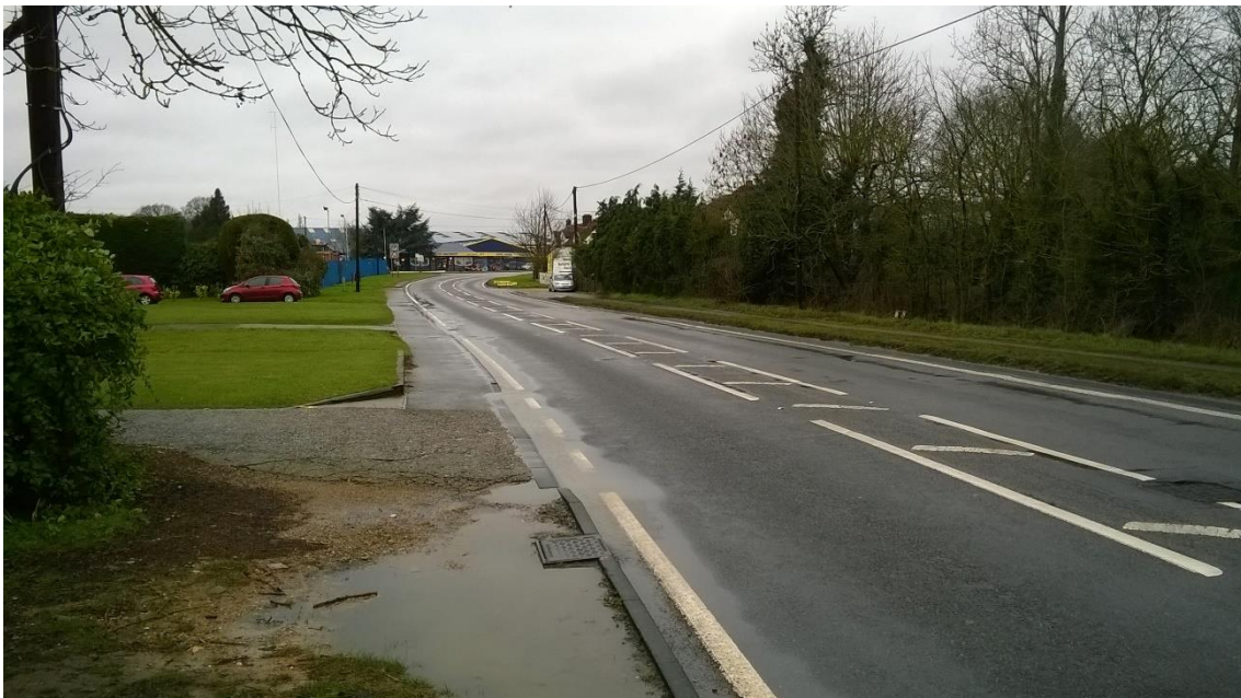
B1019 Maldon Road looking towards No.1 Little Mill Cottages and Ernest Doe & Sons yard, west bound (Gully 5 and catch pit 3 on CCTV survey are shown in the foreground).
